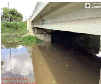
Puente Tupé PR 11+652 17/10/2023 11:49:23 GMT-05:00
