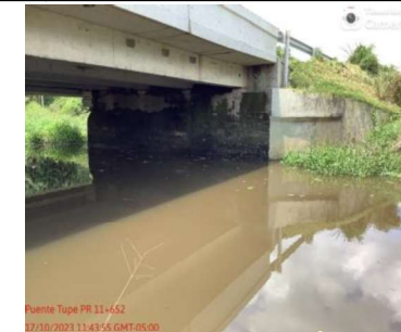
Puente Tupé PR 11+652 17/10/2023 11:53:55 GMT-05:00
