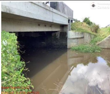
Puente Tupé PR 11+652 17/10/2023 11:52:58 GMT-05:00
