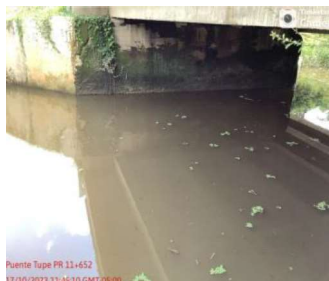
Puente Tupé PR 11+652 17/10/2023 11:46:10 GMT-05:00
