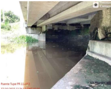
Puente Tupé PR 11+652 17/10/2023 11:36:17 GMT-05:00
