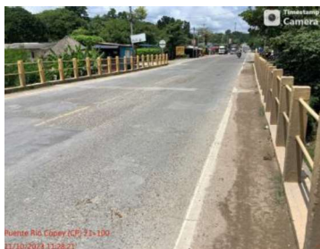
Puente Rio Copey (C) 32+100 11/10/2023 11:08:21
